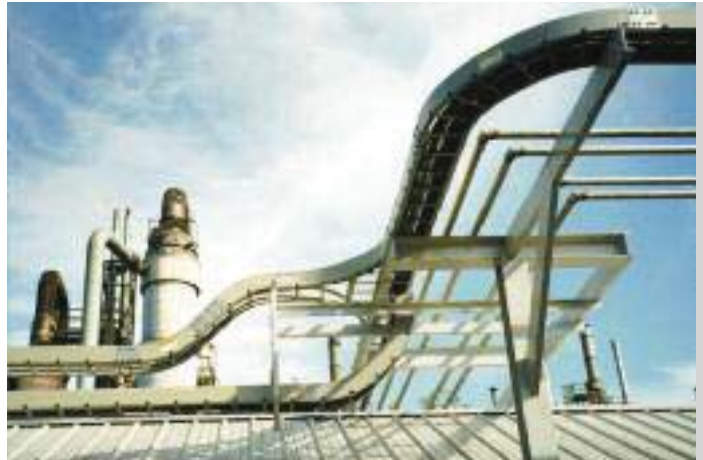
Horizontal and vertical drops, exterior installation
